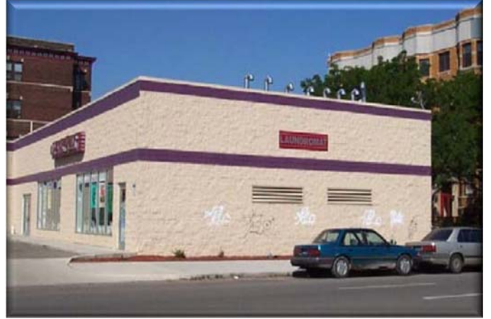
Retail building with a blank wall facing a street. The blank wall is abutting a sidewalk with openings used for ventilation grilles instead of storefront and entryways.
