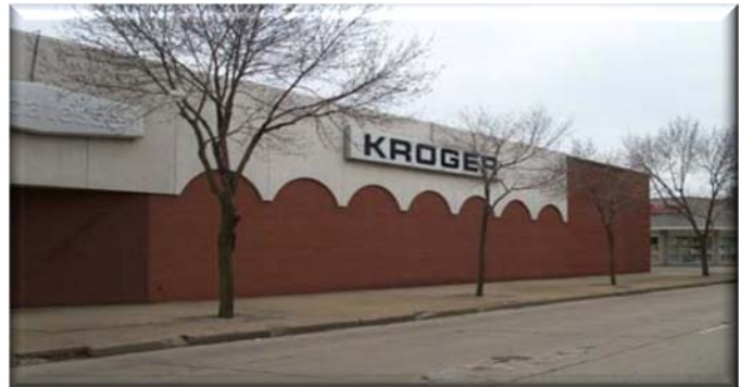
Store has attempted to enhance the blank wall by applying arches on the brick surface in a different material and color and placement of sign. Unfortunately, this side is missing entryways, storefront and display windows.
