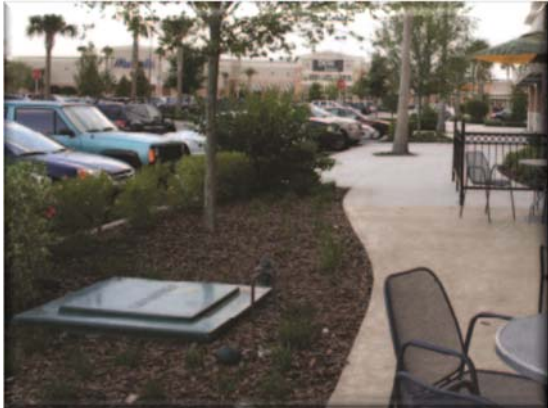
Locating utility boxes in the landscape planter prevents the installation of plant material.
