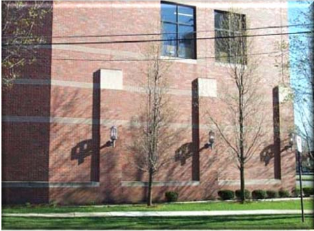
Blank wall vertical relief (brick pilaster).
