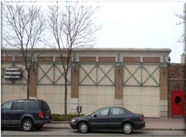
Blank wall with vertical relief (brick pilaster) and architectural metal work in between.
