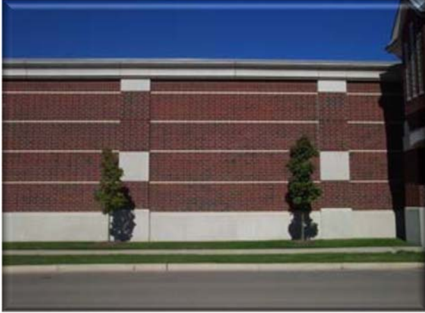
Blank wall with vertical relief (brick pilaster) and horizontal trim detail and a base.
